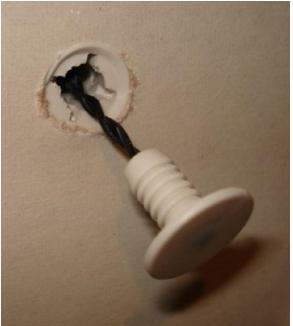
7) Use your thumb to carefully push the sensor body into the threaded outer case until the face of the sensor body is flat against the drywall.
